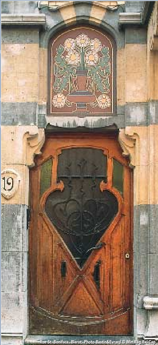
Rue St. Boniface, Blerot. Photo Bastin&Evrard © Min.Rég.Bxl-Cap
